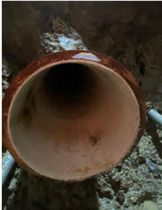
Fig 5 Lined Pipe prior to reinstatement
